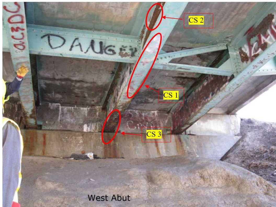
Figure 6.8 Bridge with multiple condition states
